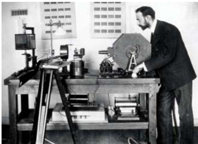
LUCIEN BULL demonstrates the high-speed camera he invented in 1903, the first to record insect flight.
