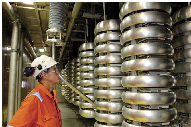
IGBT POWER: Existing IGBT-based HVDC units, like ABB’s HVDC Light system [left] and Siemens’s modular multilevel converters [right] cannot break DC current on their own.
