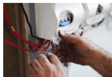
JOSEPH GIULIANO , AN ENEMALTA TECHNICIAN, INSTALLS A PLATE THAT HIDES THE WIRES CONNECTING TO NEW SMART METERS [top]. NEXT, HE PROGRAMS THE METERS WITH CUSTOMER INFORMATION [bottom left]. AS A FINAL STEP AGAINST TAMPERING, HE SEALS EACH METER WITH A BAR-CODED PLASTIC TAG [bottom right].
