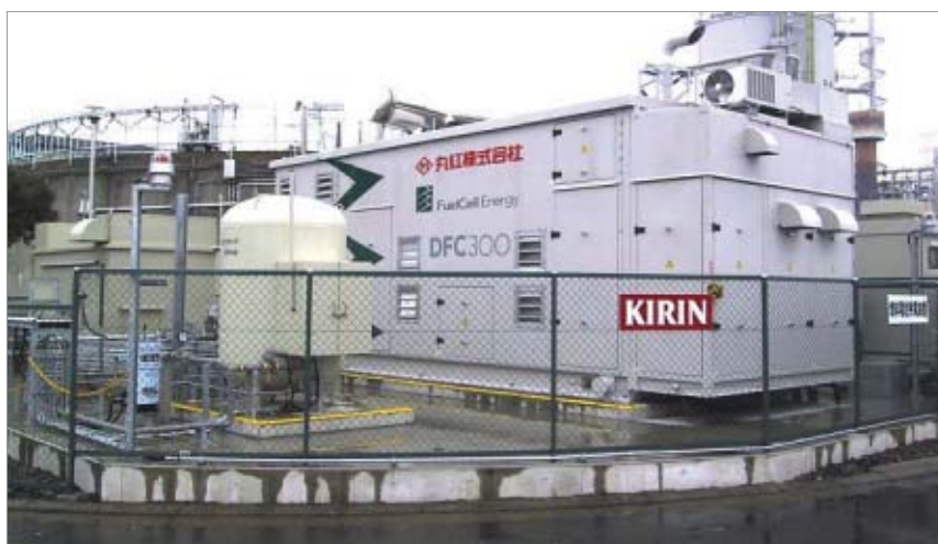
GOOD DIGESTION: A fuel cell plant powers a Kirin Brewery operation in Tokyo, which runs on its waste gases in a self-contained system. PHOTO: FUELCELL ENERGY
