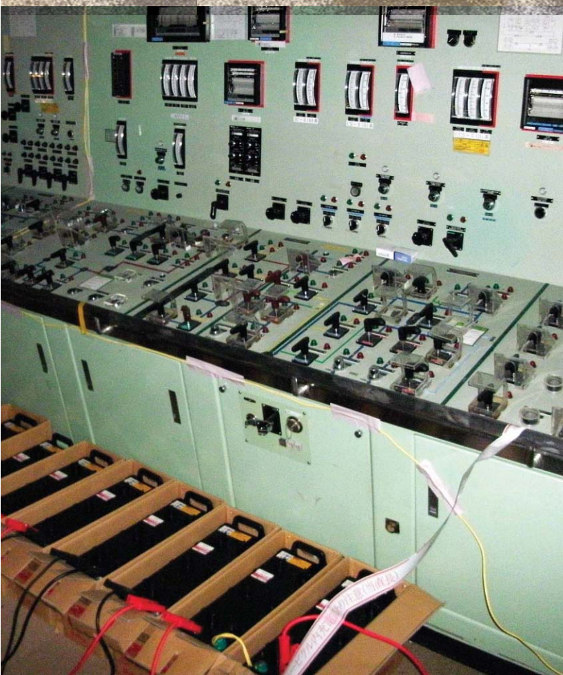
SYSTEM FAILURE: On 11 March, a TEPCO worker photographed the tsunami sweeping into the Fukushima Dai-ichi power station [top] and submerging tanks and cars [bottom]. After the plant lost electric power, operators could read instruments only by plugging in temporary batteries [left]. PHOTOS: TEPCO (3)
